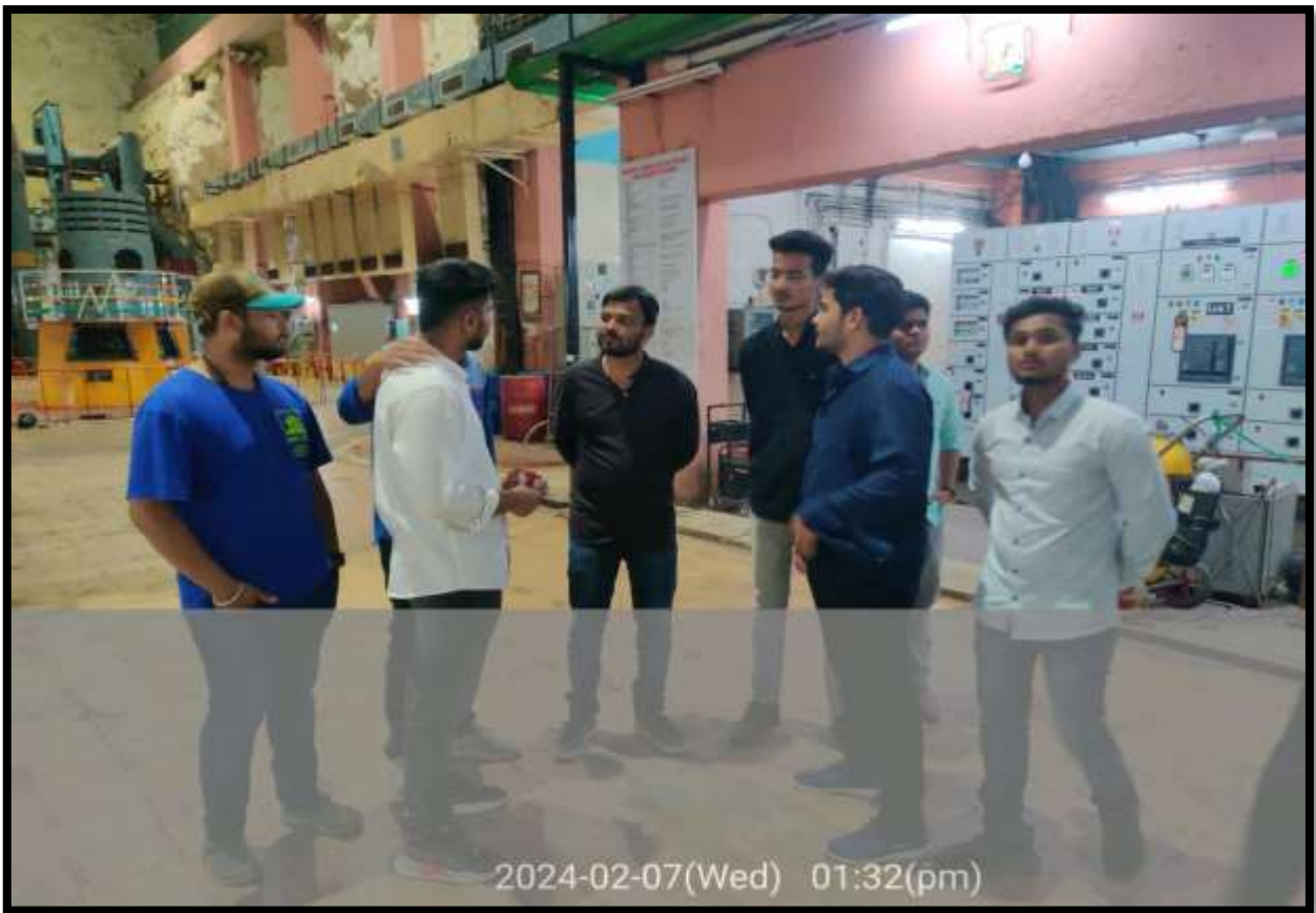
1.5 MW Hydropower Plant
