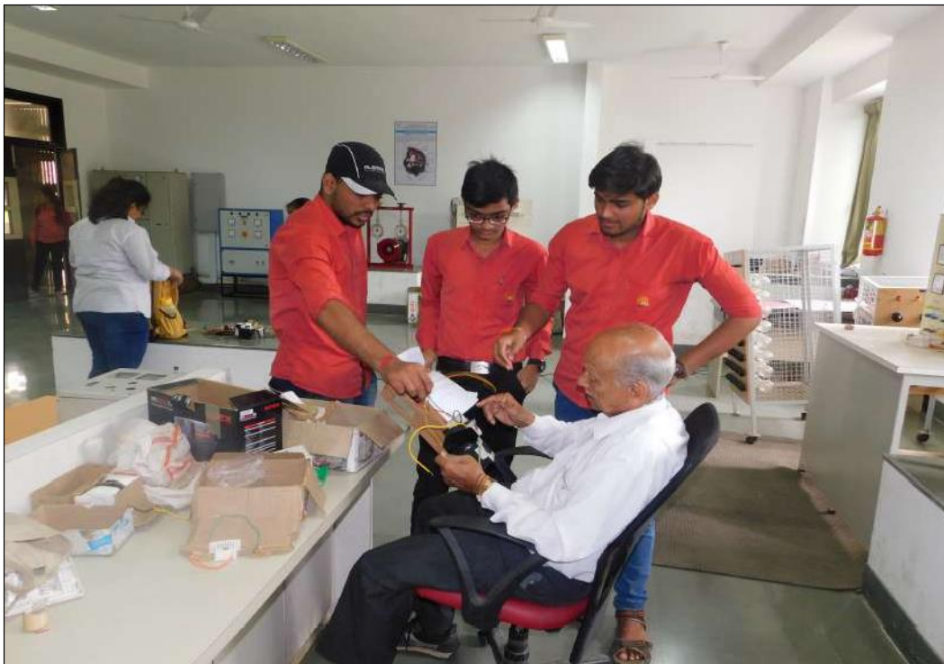
Verification of Control Panel Wiring
