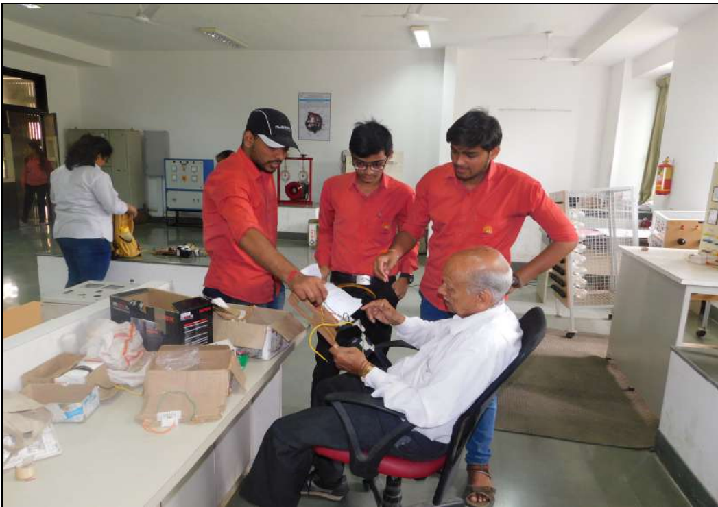
Verification of Control Panel Wiring
