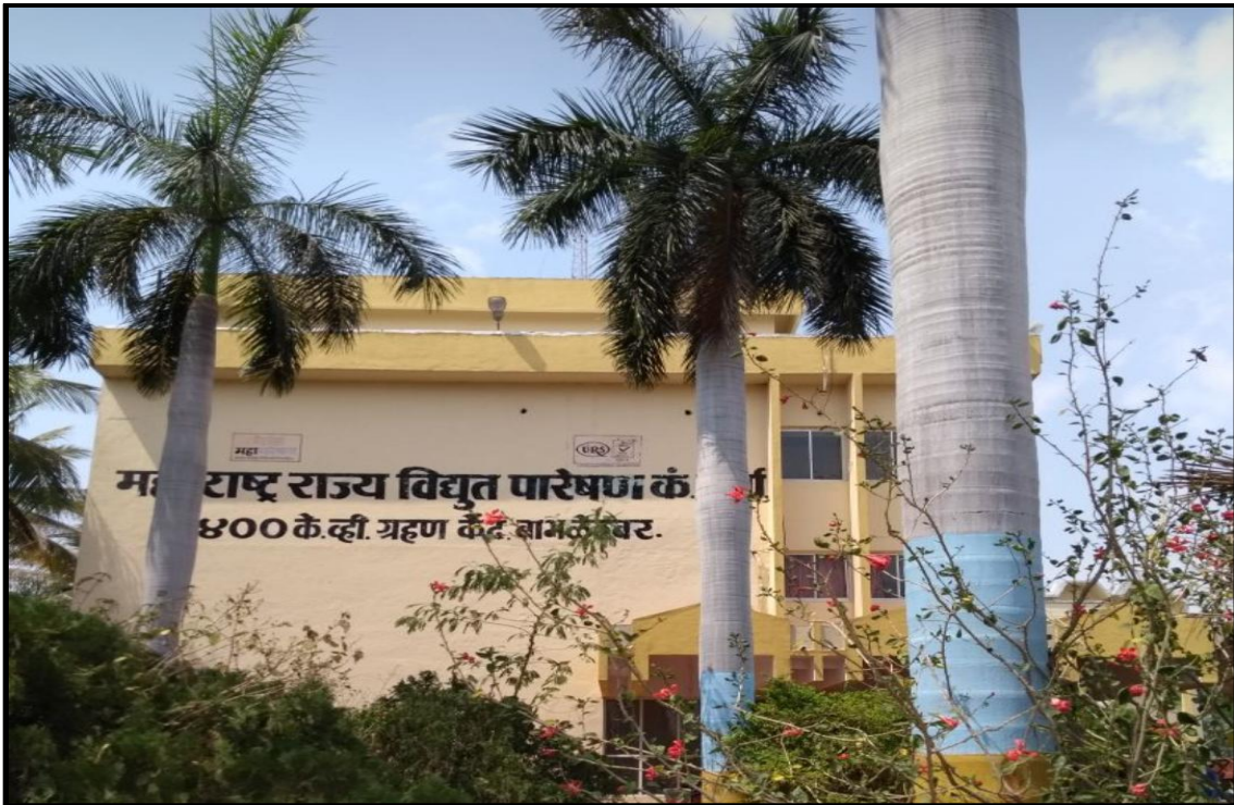
400kV Babhaleshwar Substation-Main Building
